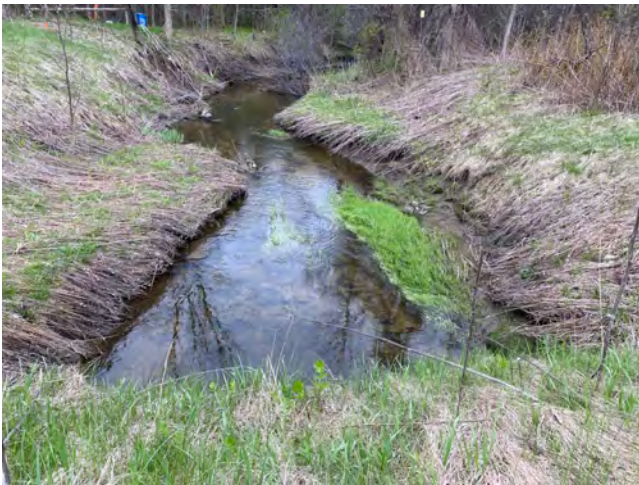
Photo 3: Site WC36; Station ET_24+364 (Elizabethtown) - Butler's Creek; Highway 401 Eastbound, facing south (downstream)
